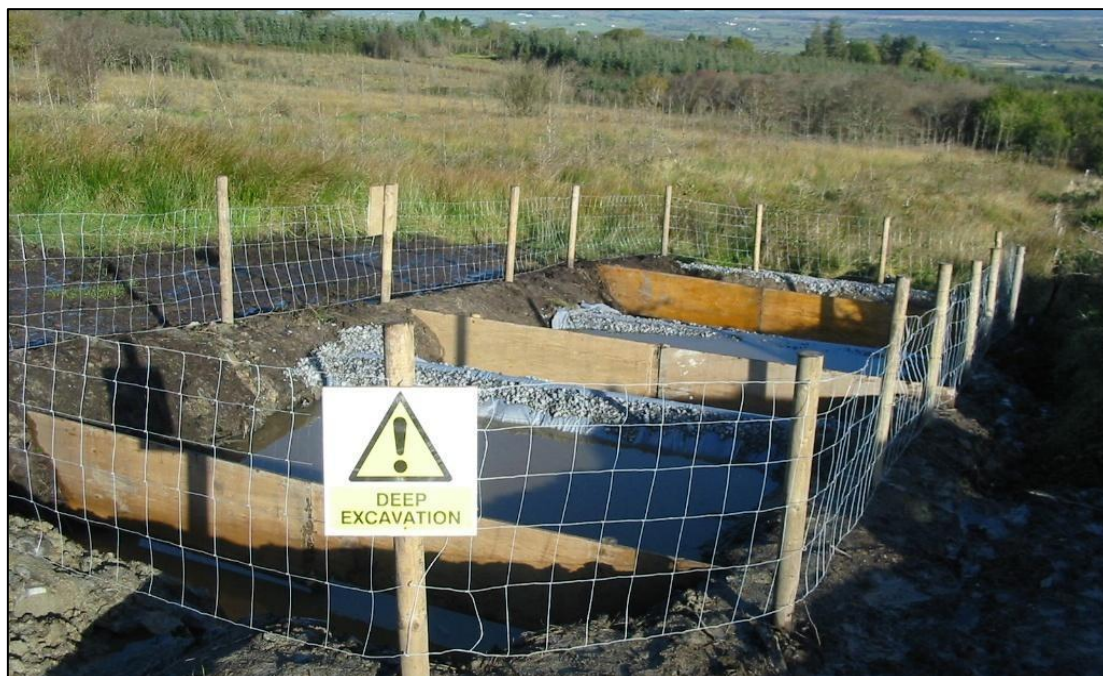
Figure 4-3: Typical Three-tiered Settlement Pond with Stone Filter
