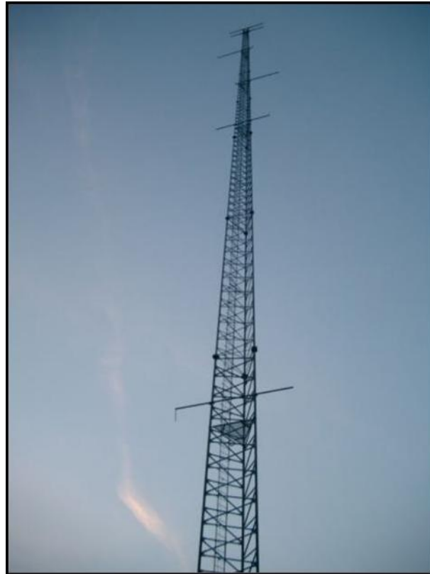
Figure 4-8: Example of a Meteorological Mast on a Wind Farm
