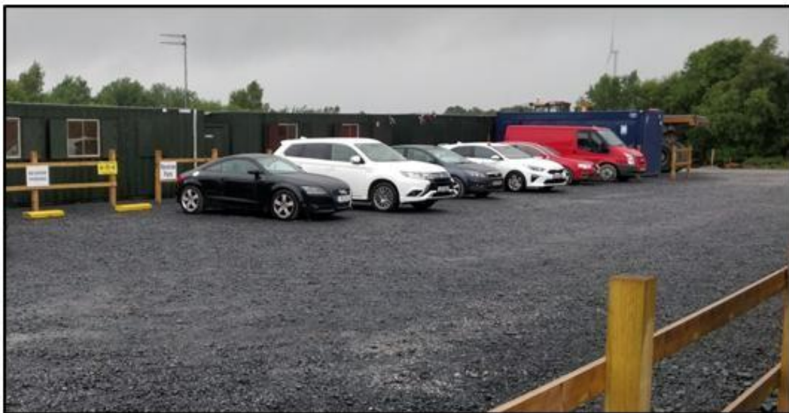
Figure 4-1: Typical Temporary Site Construction Compound on a Wind Farm
